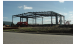
Construction in the St. Johns Industrial Park
